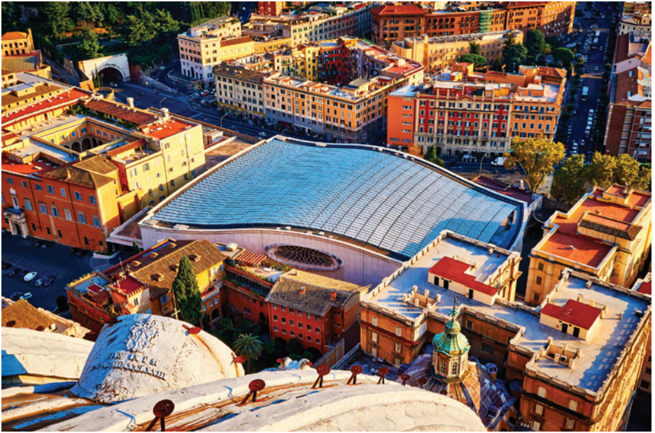
Pope Paul VI Audience Hall, viewed from the dome of St Peter's, showing the photovoltaic panel roof
